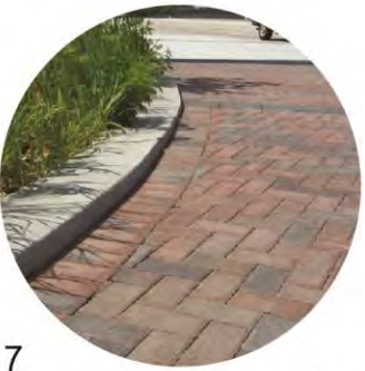
7 interlocking permeable pavers in herringbone pattern
