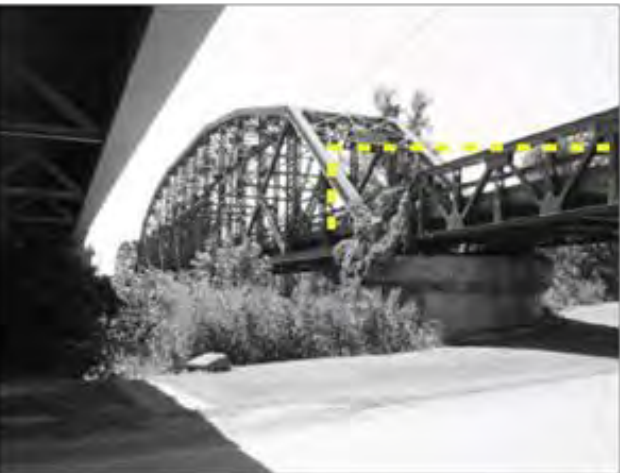
The Colorado River Bridge is a 2-part, steel truss and concrete highway bridge crossing the Colorado River on a north-south axis, Pennsylvania through truss bridge over Colorado River on Business 59 SB in Wharton Built 1930.
